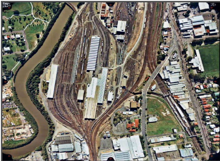
Figure 1: Queensland Rail Maintenance Depot
