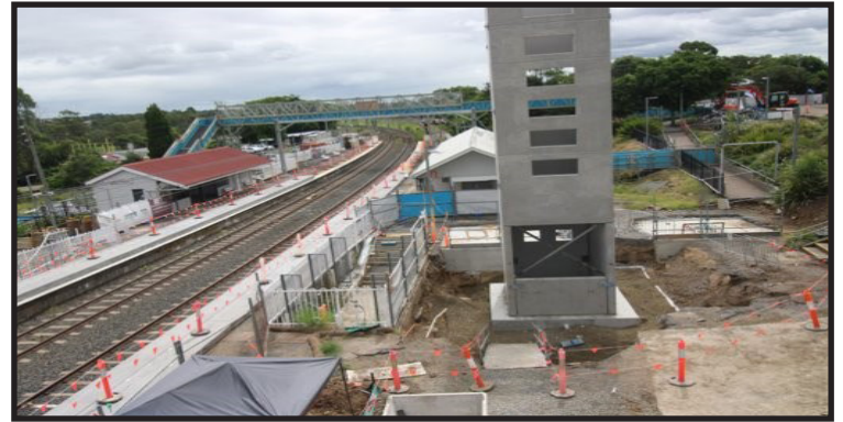
The new lift shaft and platform raising works
