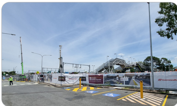
Lindum station - site separation fencing.
