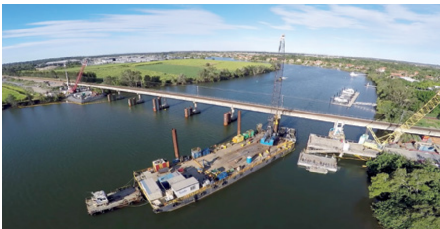
Coomera River duplicated rail bridge under construction
