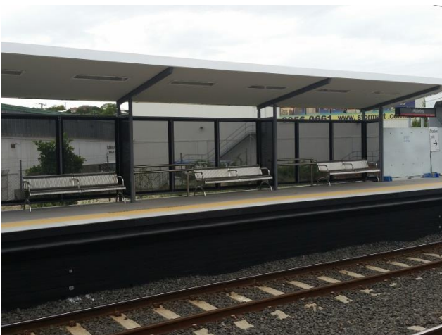
New shelter and seating, platform 1.
