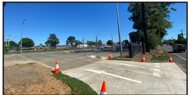
New station carpark entry from Burpengary Road
