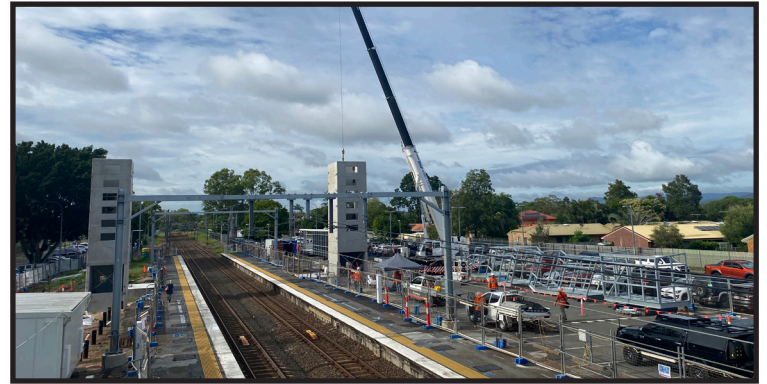
The new lift, station building and footbridge works
