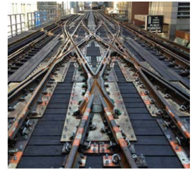
A crossover between two tracks
